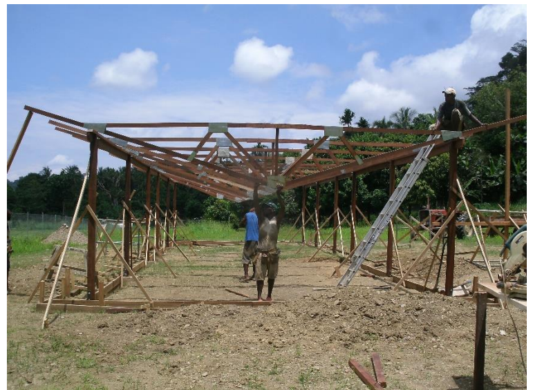
A new classroom under construction
