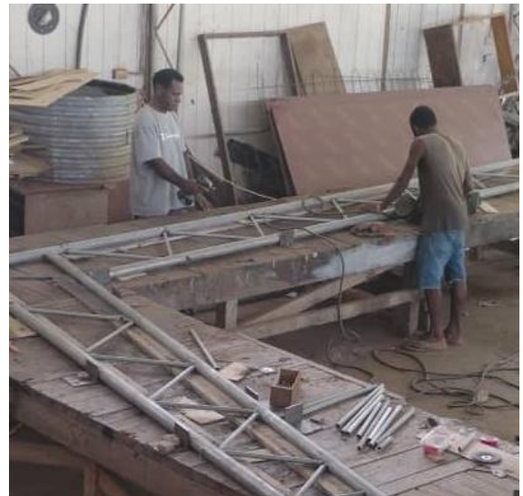
Truss preparation and welding by Ishmael and Filca at Ambunti
